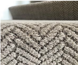
Worn stair edge from foot traffic
